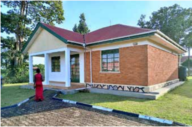
The residential house that came with the deployment.
